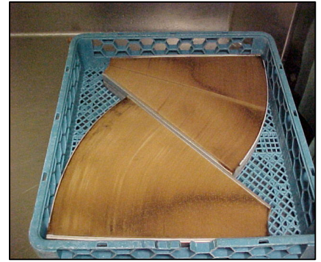
Airxchange energy transfer media ready for dishwasher cleaning.
