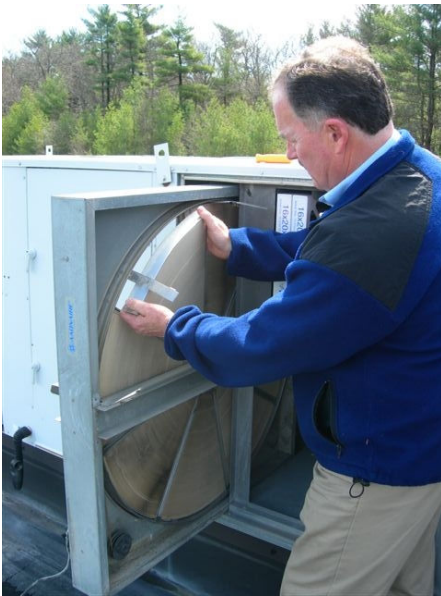
Bill Tierney, Airxchange Service Manager, demonstrates the easy segment removal on an HVAC system similar to those used by Applebee's.
