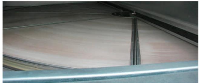
Installed in the school’s rooftop HVAC unit, the Airxchange ERV wheel dramatically reduces the cost of conditioning outside air (OA) by recovering and recycling energy from exhaust air, significantly reducing the OA (and total) load on the HVAC system.
