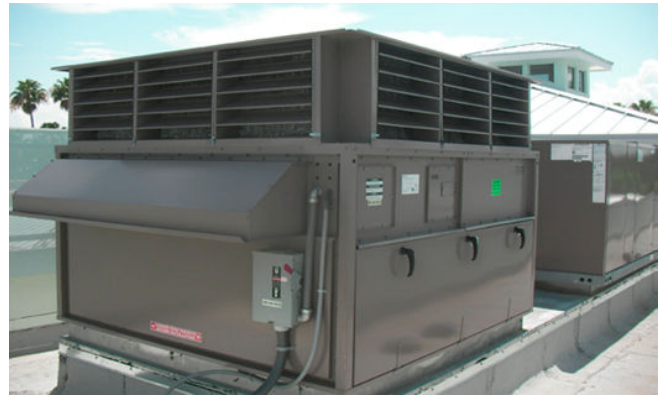
Because ERVs reduce the outside air load on the HVAC system, the rooftop unit at Turtle River is about half the size it would have been without an Airxchange wheel.
