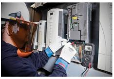
Variable-frequency drives (VFDs) have helped to reduce the number of motor failures that are the result of overheating and voltage irregularities. (Photo courtesy of Flir Systems Inc.)
