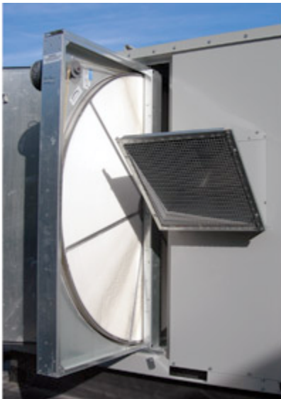
Airxchange energy recovery wheels installed at PCTA help achieve energy-savings goals.
