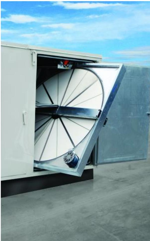
**An Airxchange energy recovery wheel is attached to a sliding cassette for easy access to the wheel. The wheel's segmented design allows for easy cleaning or segment replacement, for optimal performance over the life of an HVAC system.**
