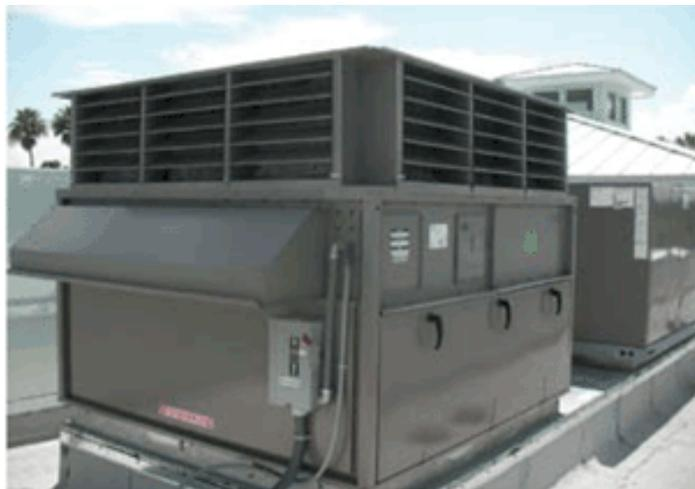
**Because the energy-recovery-ventilation (ERV) wheel reduces the outside-air load on the HVAC system, mechanical consultants were able to recommend a rooftop unit about half of the size of the one that would have been required without ERV.**
