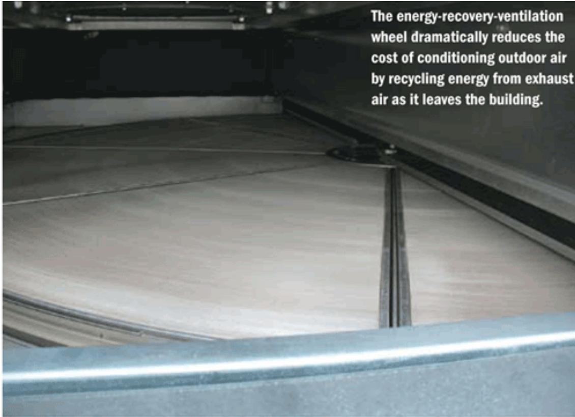
According to Eno, the system manages all of the school's outside-air ventilation, conditioning the air and feeding it into the returns of all of the air handlers. The air handlers are part of a buildingwide variable-refrigerant-flow system that modulates the refrigerant flowing through the coil. This maintains desired humidity without overcooling the building and prevents the coil from icing up.
