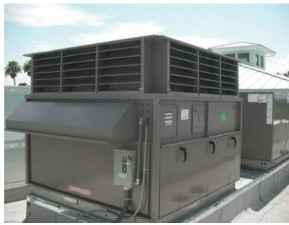
***Because the Airxchange energy recovery ventilation wheel reduces the outside air load on the HVAC system at the school, mechanical consultants recommended a rooftop unit about half the size of the one that would have been required without ERV.***
