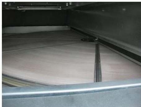
***The Airxchange ERV enthalpy wheel installed in the school's rooftop HVAC unit dramatically reduces the cost of conditioning outdoor air by recycling energy from exhaust air as it leaves the building, significantly reducing the OA (and total) load on the HVAC system.***
