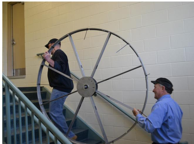
by each of the failed energy recovery wheels, which were placed into the units before the initial system installation. The cabinet door was significantly smaller than the wheel itself, making the removal of the existing wheel and the installation of a replacement more difficult. The small door also blocked “slide out” access that enables a technician to remove the wheel from the cabinet to easily perform inspections, cleaning, or repairs.
