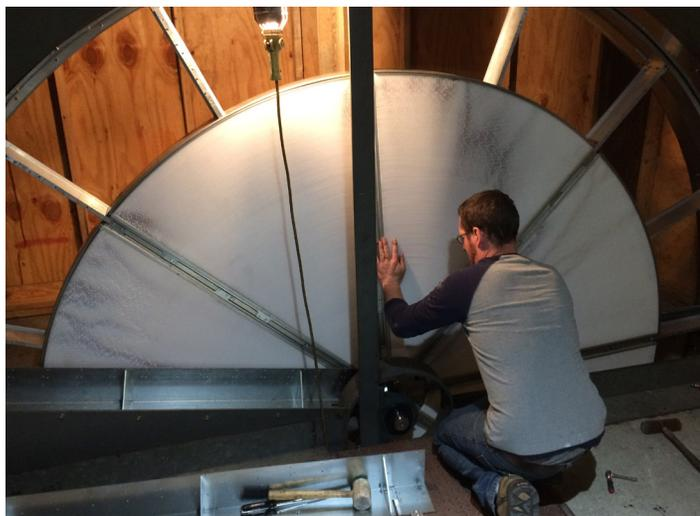
Airxchange provided a fully segmented energy transfer media that can be easily removed and cleaned. The unique design allows the entire wheel and cassette frame to be carried into the mechanical room in manageable pieces for reassembly inside of an AHU cabinet.
