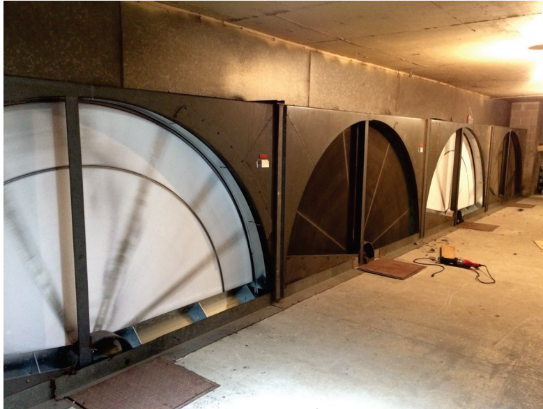
Upgrading old, uncleanable aluminum wheels with Airxchange's fully cleanable and segmented polymer wheel.
