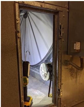
*Airxchange’s unique and practical hygienic wheel design makes it easy to remove and clean the energy transfer media outside the air-handler unit.*
