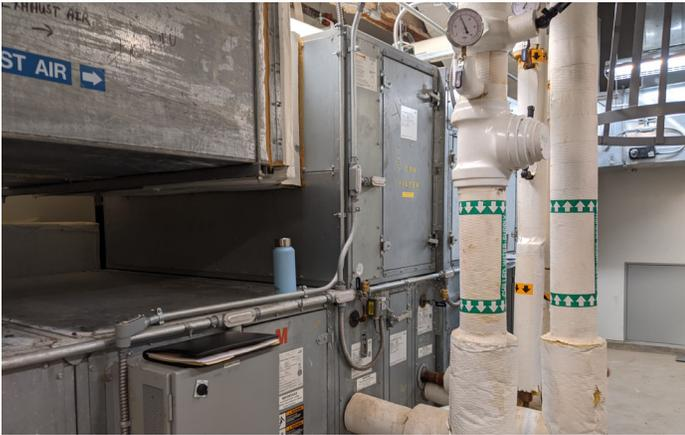
Once in the mechanical rooms, the wheels were assembled in the air handlers without interrupting the critical operations of the facility, and then powered on to return the ventilation system to an energy saving asset for the Veterans Home. To enable optimal performance over the lifetime of the new wheels, Airxchange provided hands-on instruction to the facility staff to develop a preventative maintenance strategy to help the facility maintain optimal operational efficiency.
