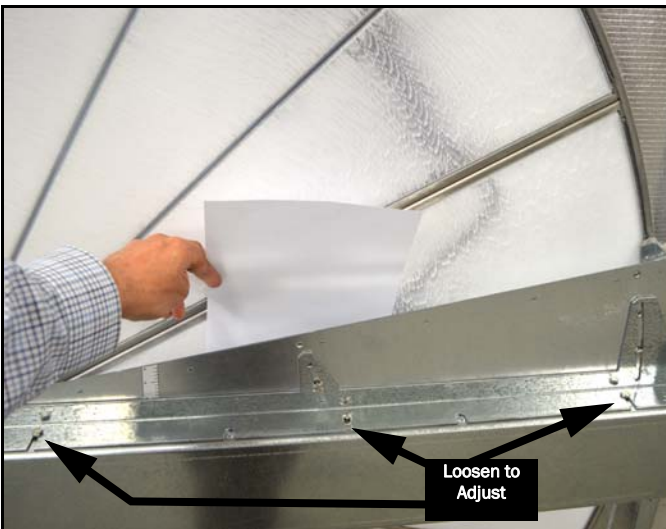
Figure 10 Check purge seal and adjust (if necessary).
